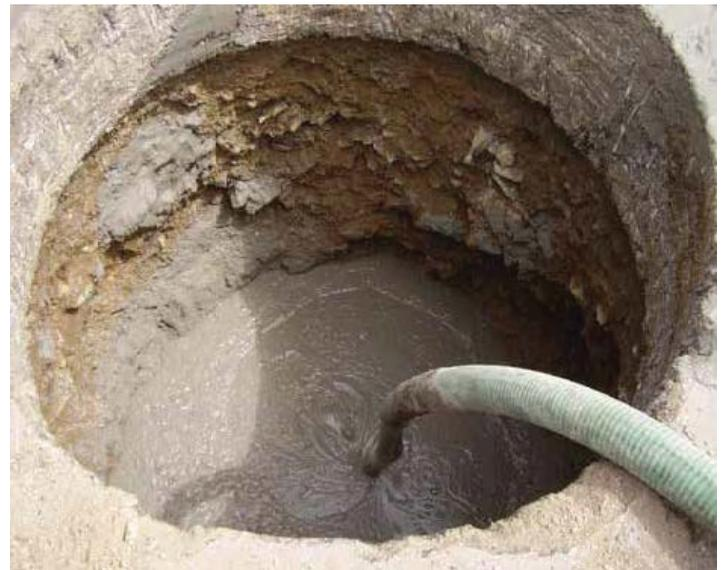
36-39 pcf Low-Density Cellular Concrete with a 2" slump and minimum strength of 80 psi placed in single lifts of up to 20'
