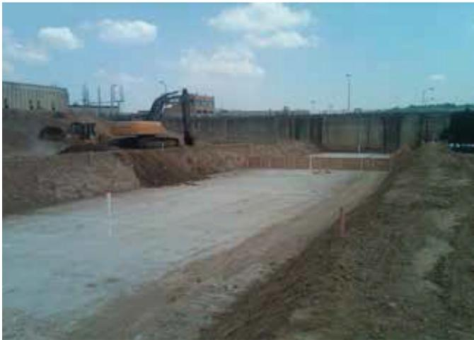
Excavation and placement of new concrete slab over existing outfall conduit
