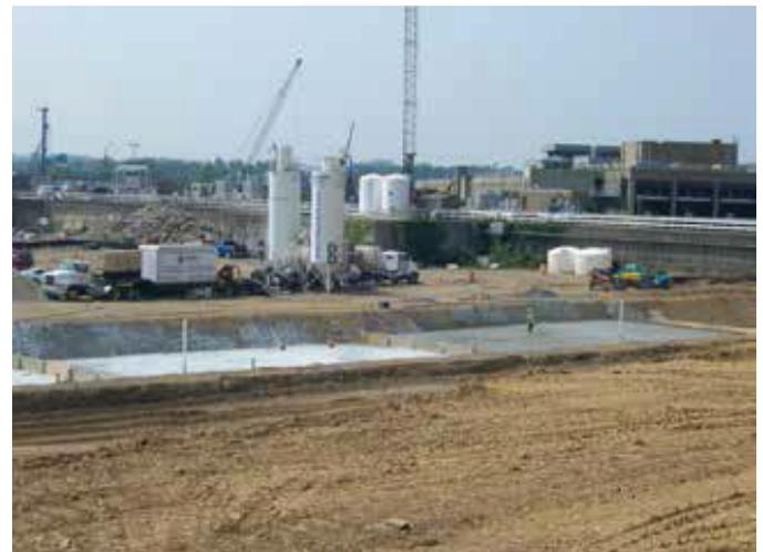
Placement of Low-Density Cellular Concrete backfill to reduce load on existing conduit structure
