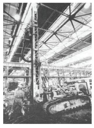
The repair plan included the installation of micropiles to stabilize the maintenance building, Low-Density Cellular Concrete (LDCC) to fill existing voids under the floor slab and several new structures and equipment.
