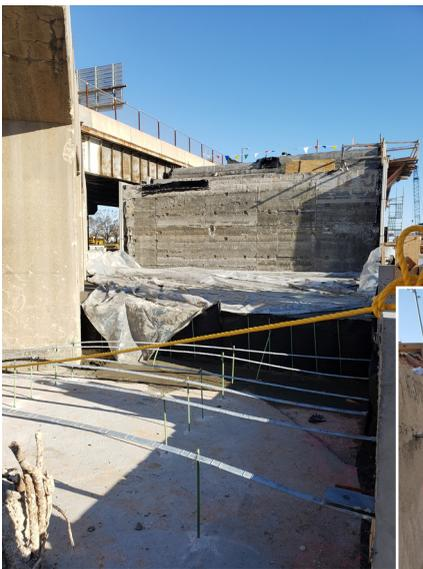
Given these challenges, the design team knew this project required a backfill product light weight enough to reduce the load placed on the soft subsoils, and strong enough to provide long-term stability and eliminate the need for compaction. With this in mind, they chose to use AERLITE-iX™, a non-permeable, Low-Density Cellular Concrete (LDCC) product manufactured by Aerix Industries™, to complete the backfill of the mechanically stabilized earth wall.
