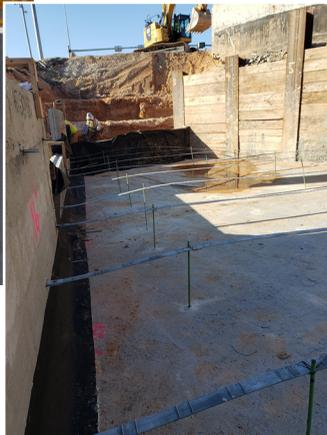
A three-person crew from Geo-Cell Midwest, LLC installed more than 20,000 cubic yards of LDCC at a density of 25-35 pcf per project specifications. The crew used 30-inch lifts to complete the installation, placing the LDCC over previously driven micropiles with a slab of traditional concrete. Due to the cold winter temperatures, the Geo-Cell Midwest crew used special care in mixing the LDCC, making sure to adjust the mixture as needed to facilitate a speedy and effective installation.
