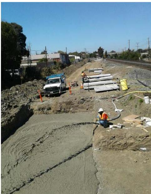
This ongoing project comprises a number of smaller projects and steps within the construction process—this includes lowering multiple road surfaces; building approximately one mile of mechanically stabilized earth (MSE) wall; constructing five bridges; constructing elevated railway tracks; and designing a new, elevated train station.
