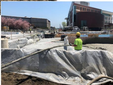
The manufacturing and installation firm inTerra installed a total of 6,000 cubic yards of Aerix's AQUAERIX PLDCC across the UMass campus to remediate soft soils and enhance the structural stability of multiple facilities. Because it is highly flowable, AQUAERIX provided a quick and easy application, enabling this project to be completed during the summer months before the influx of new and returning students in the fall semester.
