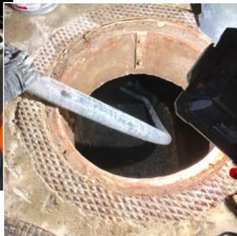
The installation crew from SERD Construction pumped 40 cubic yards of 30-pcf AERLITE-iX into the two abandoned vaults, using three lifts for each vault. During this installation, the SERD team weighed the AERLITE-iX foam daily and regularly tested the wet density of the installed product to ensure the highest quality performance.
