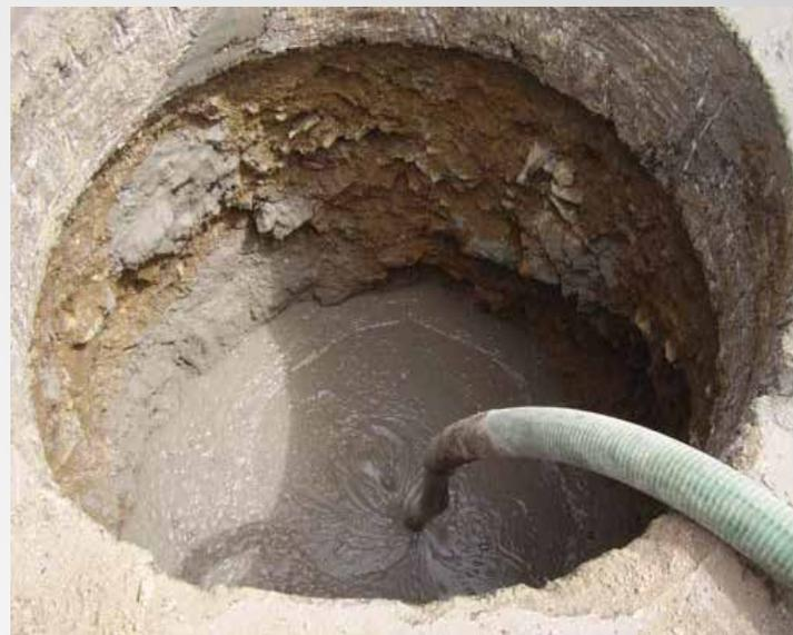
36-39 pcf low-density cellular concrete with a 2" slump and minimum strength of 80 psi placed in single lifts of up to 20'
