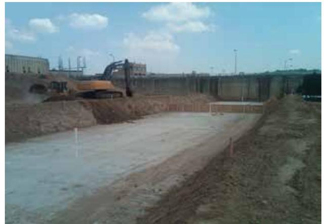
Excavation and placement of new concrete slab over existing effluent outfall conduit
