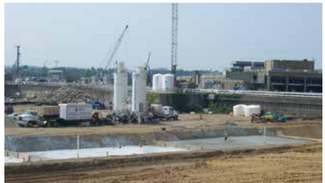
Placement of low-density cellular concrete backfill to reduce load on existing conduit structure. Material was produced on site using a mobile batch plant, silo and foam generating equipment
