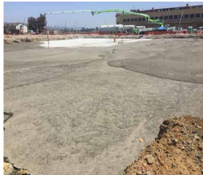
Aerix's Aerlite™ low-density cellular concrete (LDCC) was chosen for this application because it provided these characteristics while also offering quick-and-easy installation. In May 2017, the installation crew from Flashfill Services and The Conco Companies installed 17,000 cubic yards of Aerlite at a rate of 180 CY per hour (avg 1,250 CY per day) to support 45,000 square feet of structure, using in-line foam injection to pump the concrete for distances of more than 1,000 feet.
