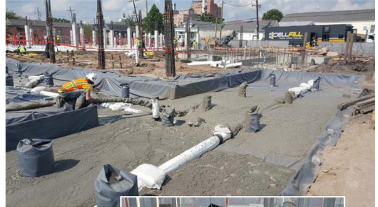
The four-person installation crew from Oklahoma-based contractor CellFill placed a total of 420 cubic yards of 30-pcf Aerix's AQUAERIX™ PLDCC in less than one day. Once the PLDCC was placed, an additional geomembrane material was installed before the main slab of the building's foundation was laid.
