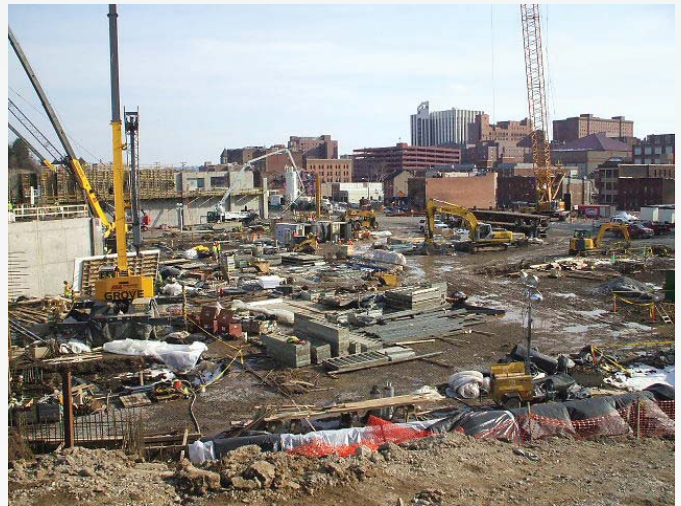
The congested site and winter weather presented challenges throughout construction
