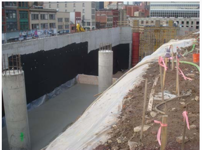
Cellular Concrete used for load reducing backfill adjacent to the foundation walls
